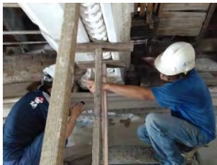
Wood Beams Inspecting
