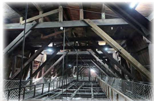
◆屋頂木構架與檢修通道(貓道)
