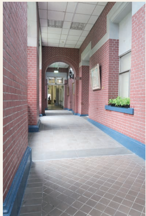
Figure 2-33 The first-floor corridor ramp.
