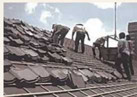
Putting a new cover in place on the roof
