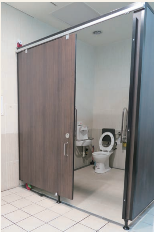
Figure 2-32 Addition of accessible toilet facilities.
