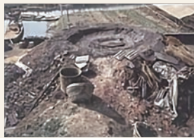
Mixing and blending soil material
