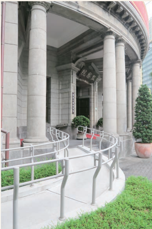
Figure 2-34 The main entrance's accessible access ramp.
